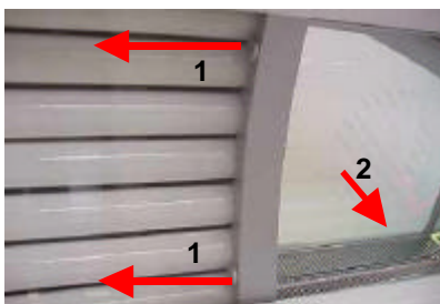
Fig. 5.8 Dismantling the tube covering
