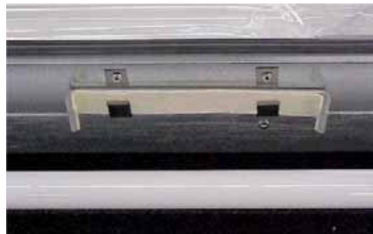
Illustr. 5-5 Suspension of the base pane
